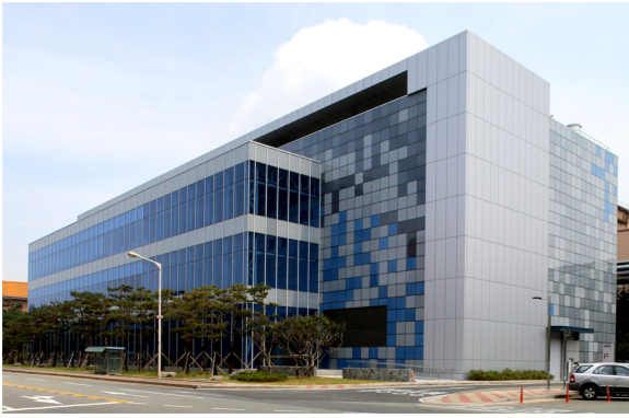
Fig. 2. Different colored BIPV installed on a building[8].
