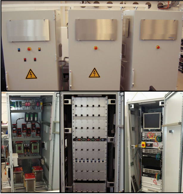
Fig. 30. Cabinets for components interfacing SMs with ac and dc sides (left), SMs (middle), and control hardware (right).
